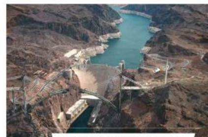
■ The Hoover dam (US) was the highest dam in the world when it was finished in 1935.
